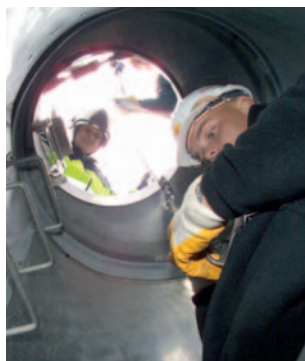
Supervising confined space entry
